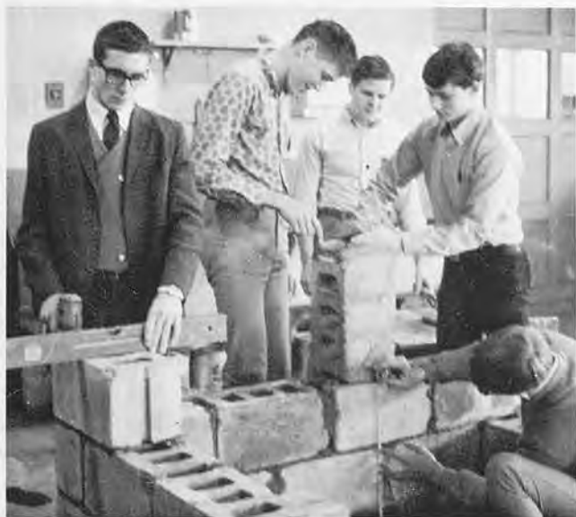
DURING THE STUDY OF A UNIT ON MACHINERY and concrete, Ag III students Tim Joyce, Mike Gaffney, Chet Rinehart, Jim Ashline, and Mark Gasser learn the basic principles of laying up a concrete block wall.
