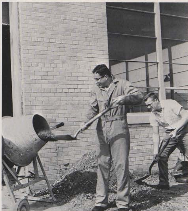
In a unit on concrete and masonry students are taught to mix concrete. John Wegert and Melvin Holton are getting some practical experience in mixing concrete.
